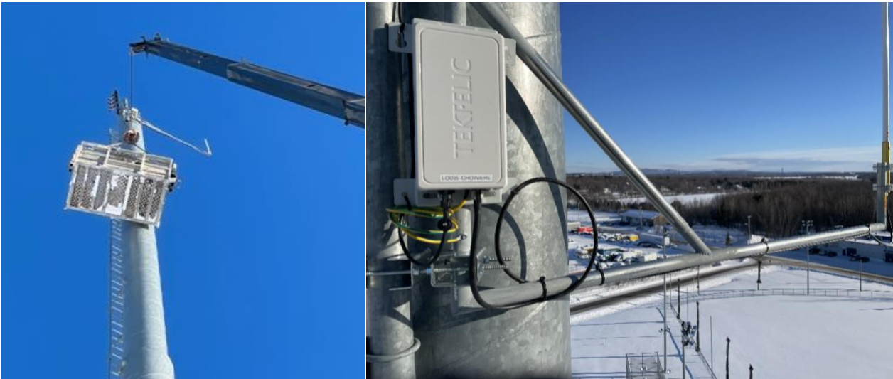
Figure 2: LoRaWAN Gateways Deployment at 110 foot Telecom Tower using a Boomer Crane
